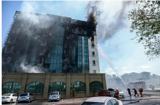
The EPF building at Jalan Gasing caught fire around 11.30am in Petaling Jaya February 13, 2018.
